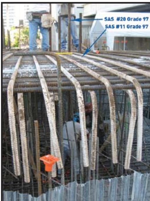
The image to the left shows the SAS #11 thread bars for rebar matting in the foundation of the Epic Tower project, Miami, FL. The #11 thread bars were bent to 90° using a conventional bending machine.
