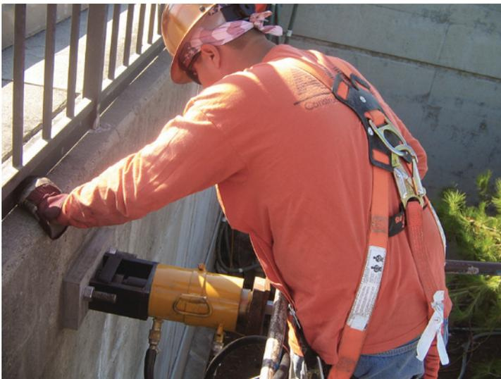
Seismic retrofit of pedestrian overcrossing using SAS Rock Bolts
